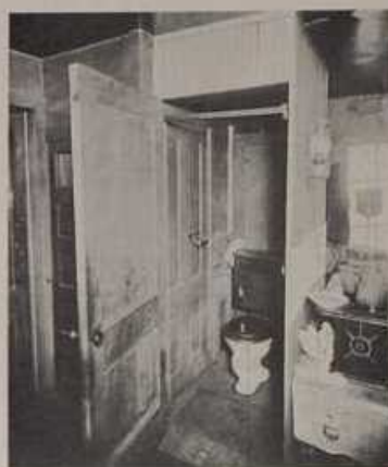
Partitioned toilet in kitchen. Open at top. No other ventilation.
