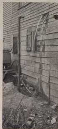
Sink drains through side of house into yard.
