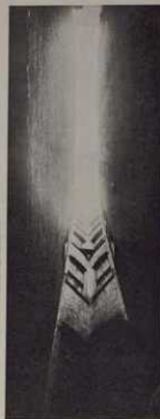
Looking up an air shaft which provides light and ventilation for 32 rooms.
