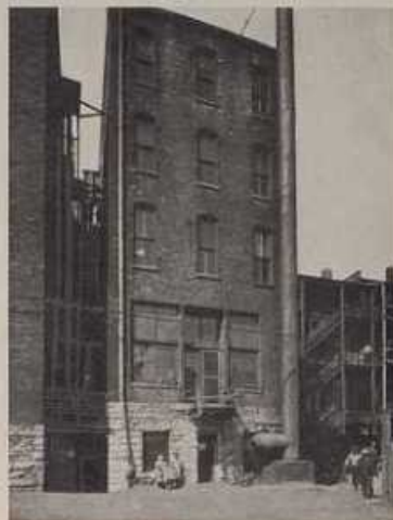
Airshaft and court showing elevator, fire escapes and garbage chutes.
